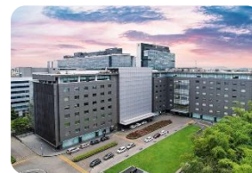
Panchshil Tech Park, Pune 0.22 MSF
